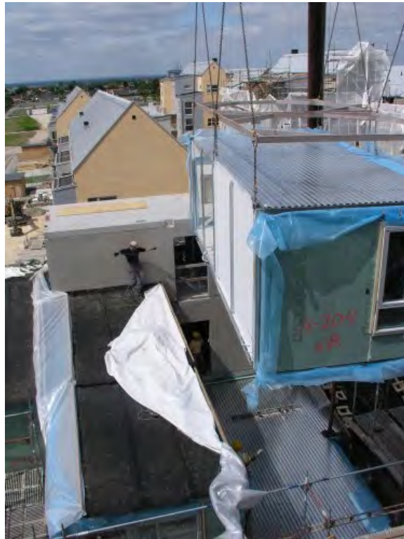
Figure 5 Assembly of modules on the construction site
