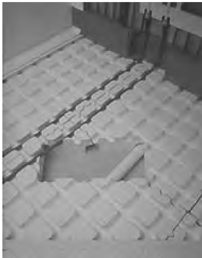
Figure 2: Matura Infill System (space reservations for ducts and services, based on modular coordination.)
