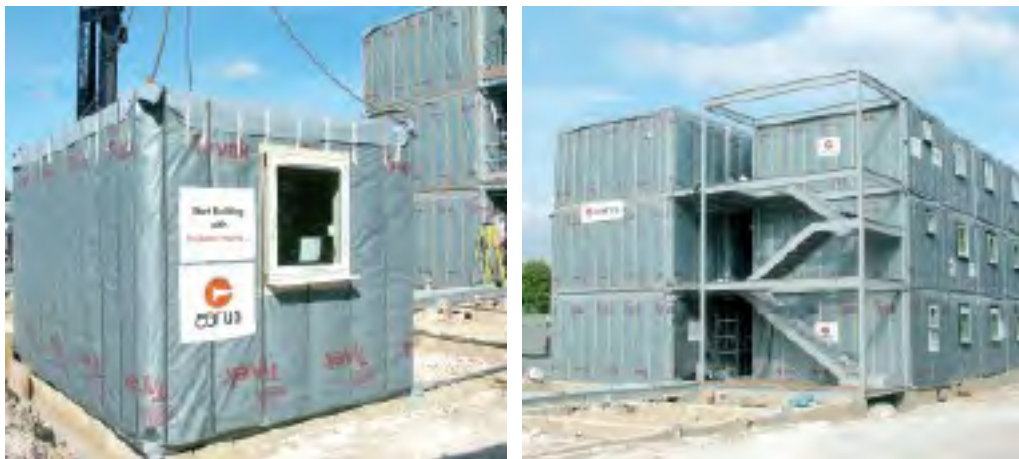
Figure 8 Prefabricated rooms put together on site.
