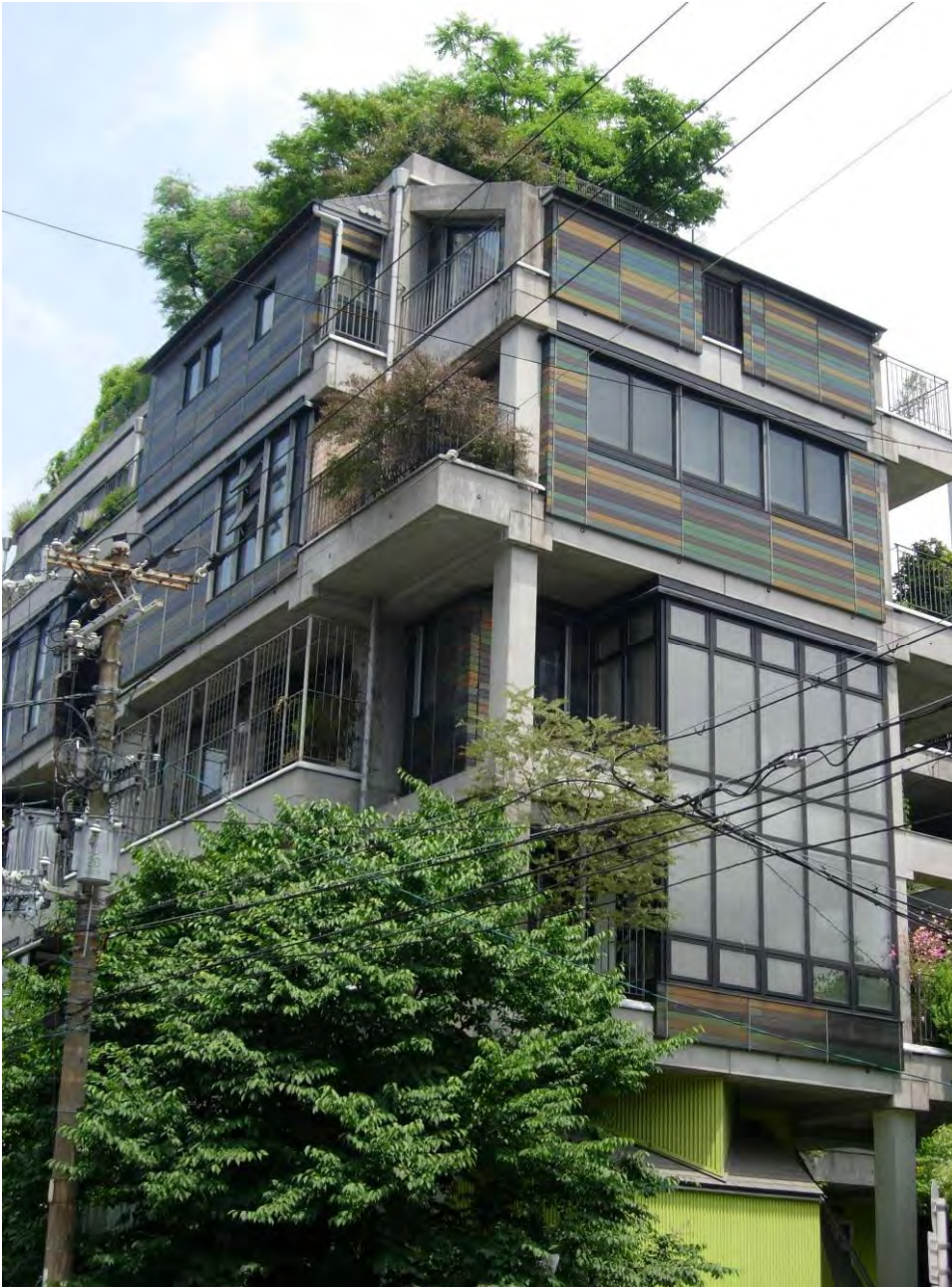
Figure 3 - The NEXT-21 prototypical flexible residential building in Osaka
